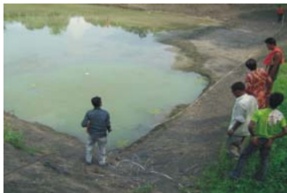
Pit measurement by Technical Assistant at worksite
